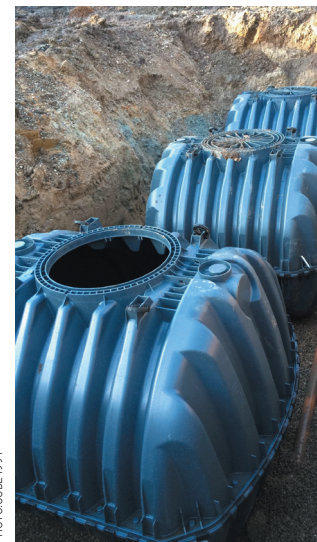
In Danbury 25,000 litre capacity tanks were placed underground to collect rainwater on an extensive project by Cube 1994
