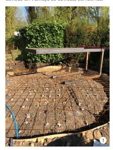
Image 1 shows the floating table during construction, created from a heavy duty box metal main frame and angle iron top frame. Box metal is used here to reduce movement once
