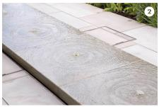
the angle iron frame is filled with a clear epoxy resin. We tested it with 127kg resting on the end of the cantilevered angle iron frame, and it only moved 5mm; when we set it into position, we offset the level to allow for the calculated load of 127kg.
